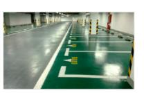
It is a surface hardening material which is ready to use, cement-based, contains corundum and spesifically
